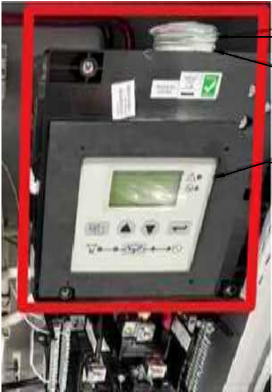
GENERATOR ALARM PANEL DETAIL
