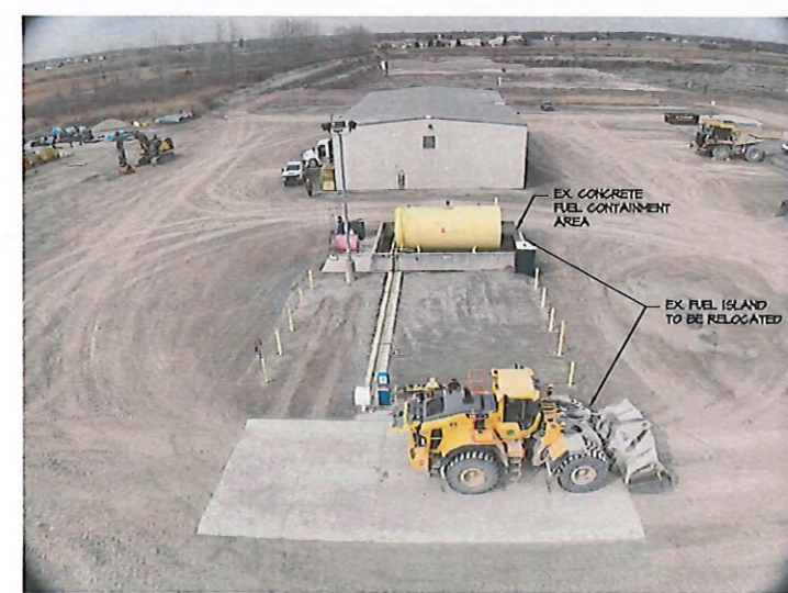
AERIAL VIEW OF EXISTING FUEL ISLAND LOCATION DRONE PICTURE TAKEN 5-25-26
